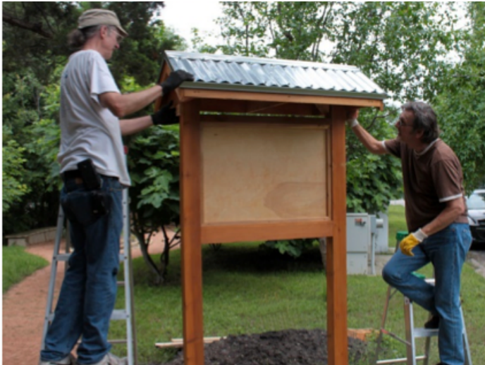
Terry Dyke and Jules Kniolek complete construction of the kiosk
